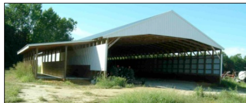
Manure storage shed. Photo courtesy of TJ Farms.
