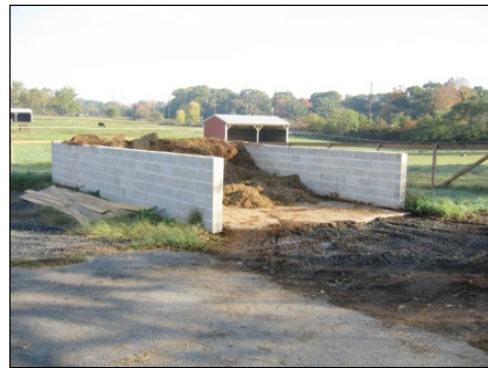
Horse manure storage area. Photo courtesy of the Livestock and Poultry Environmental Learning Center.
