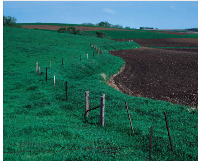
Figure 29. This ridge diversion collects runoff from water above and safely diverts it away from land that might otherwise be damaged by the runoff. Photo by Lynn Betts, USDA-NRCS.
