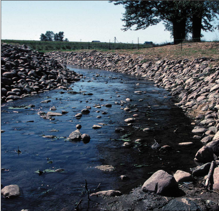
Figure 18. This stream bank has been stabilized from erosion with rip-rap. Photo courtesy of the USDA–NRCS.
