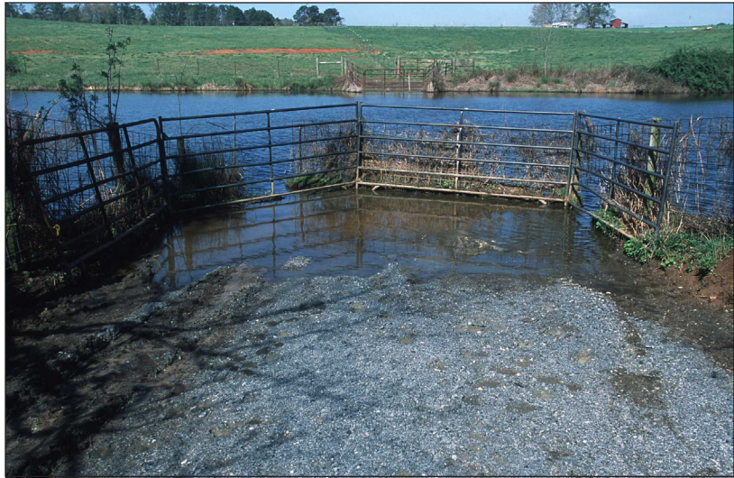
Figure 22. Example of an in-stream watering point installed on a local farm pond to prevent cattle from disturbing the adjacent riparian area. Photo by Jeff Vanuga, USDA–NRCS.
