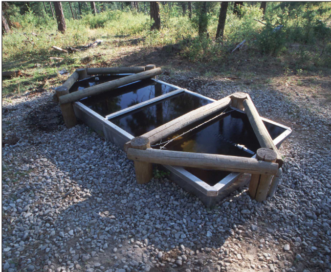
Figure 21. A water tank is an example of an area that receives heavy use. The soil surface can be protected by using geotextile materials and a layer of gravel. Photo by Gary Wilson, NRCS.
