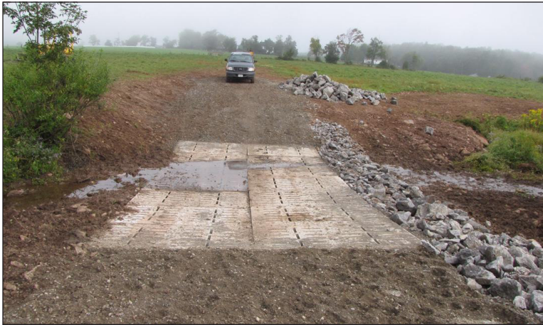
Figure 19. Hardened crossing points constructed of geotextile fabric, concrete panels, and fine gravel to facilitate cattle movement across specific points in the stream. Photo courtesy of Chenago County Soil and Water Conservation District.
