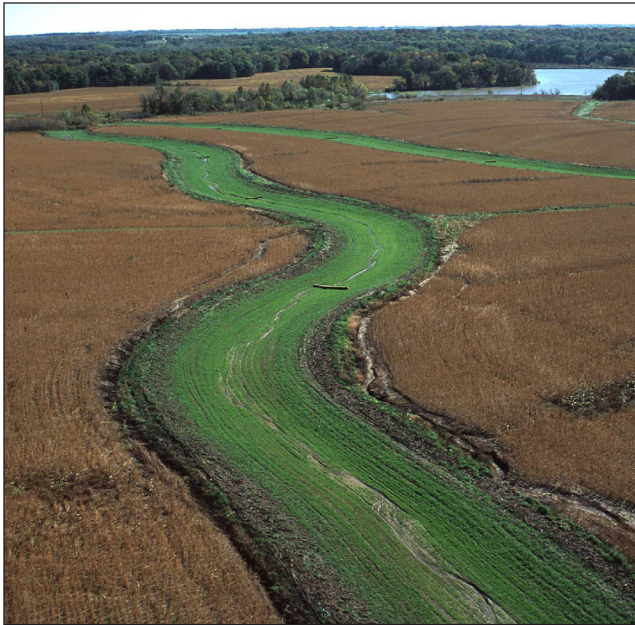
Figure 28. Grassed waterway. Photo courtesy of the USDA-NRCS.
