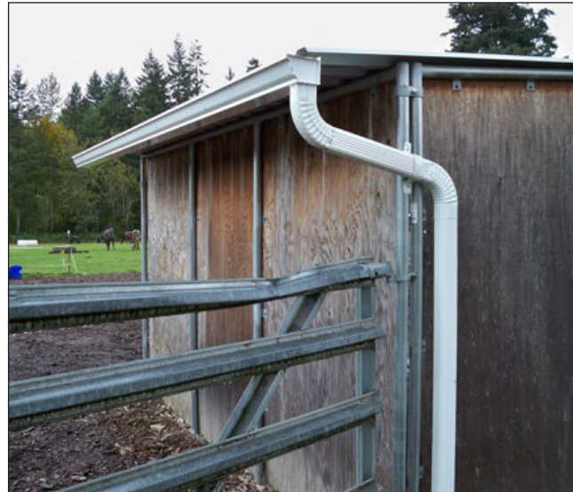
Figure 10. A roof runoff structure like the one pictured helps collect, control, and transport precipitation from roofs. Photo courtesy of the King Conservation District.
