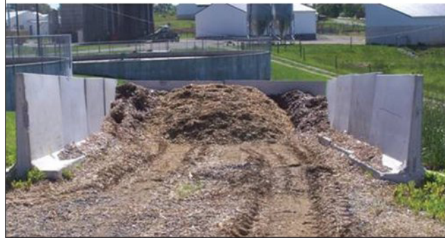
Figure 14. Bunker-type storage structure (Ogejo and Collins 2009).
