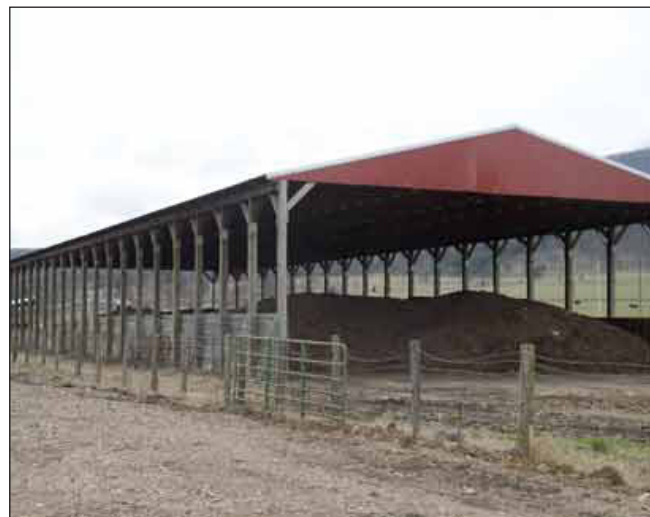
Figure 15. Poultry litter storage facility. Photo courtesy of the USDA-NRCS.
