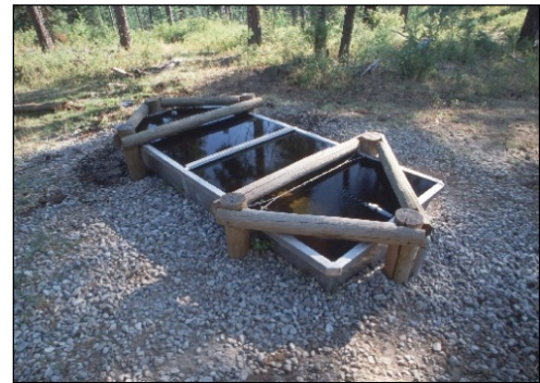
A water tank is an example of an area that receives heavy use. The soil surface can be protected by using geotextile materials and a layer of gravel. Photo by Gary Wilson, NRCS.
