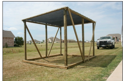
Livestock shade structure constructed of wood and a shade cloth roof. Photo by Larry Redmon.
