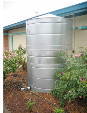
Rainwater harvesting captures, diverts, and stores rainwater for later use. Capture rainwater can then be used for a variety of different purposes including clean water for livestock. Photo courtesy of Texas AgriLife Extension.
